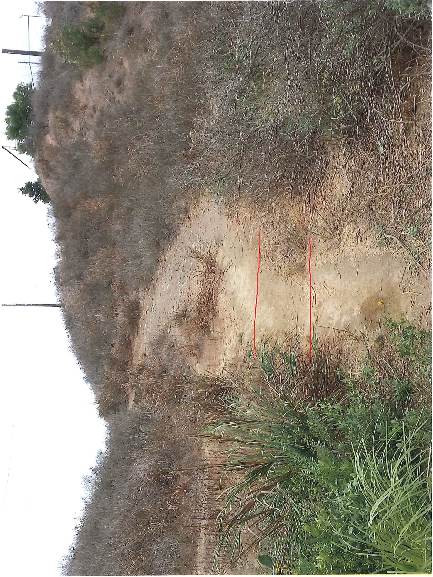
Drain marked in red and high area South of BHSO Parking lot that can be cut down so trail starts from a lower point.
