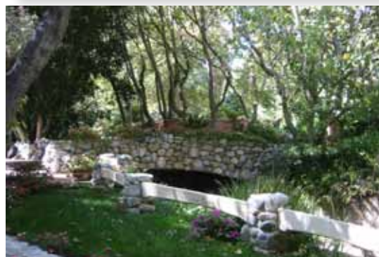
Bridge over Ramirez Creek
