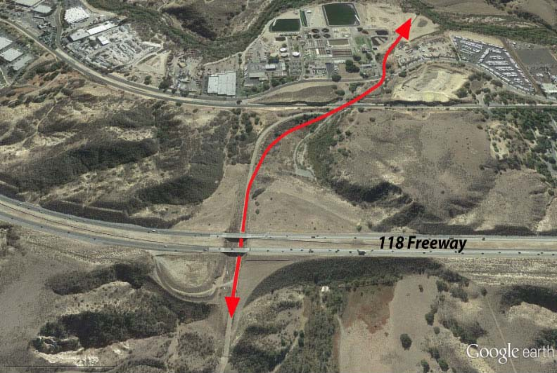
Alamos Canyon 118 Freeway Undercrossing Looking South
