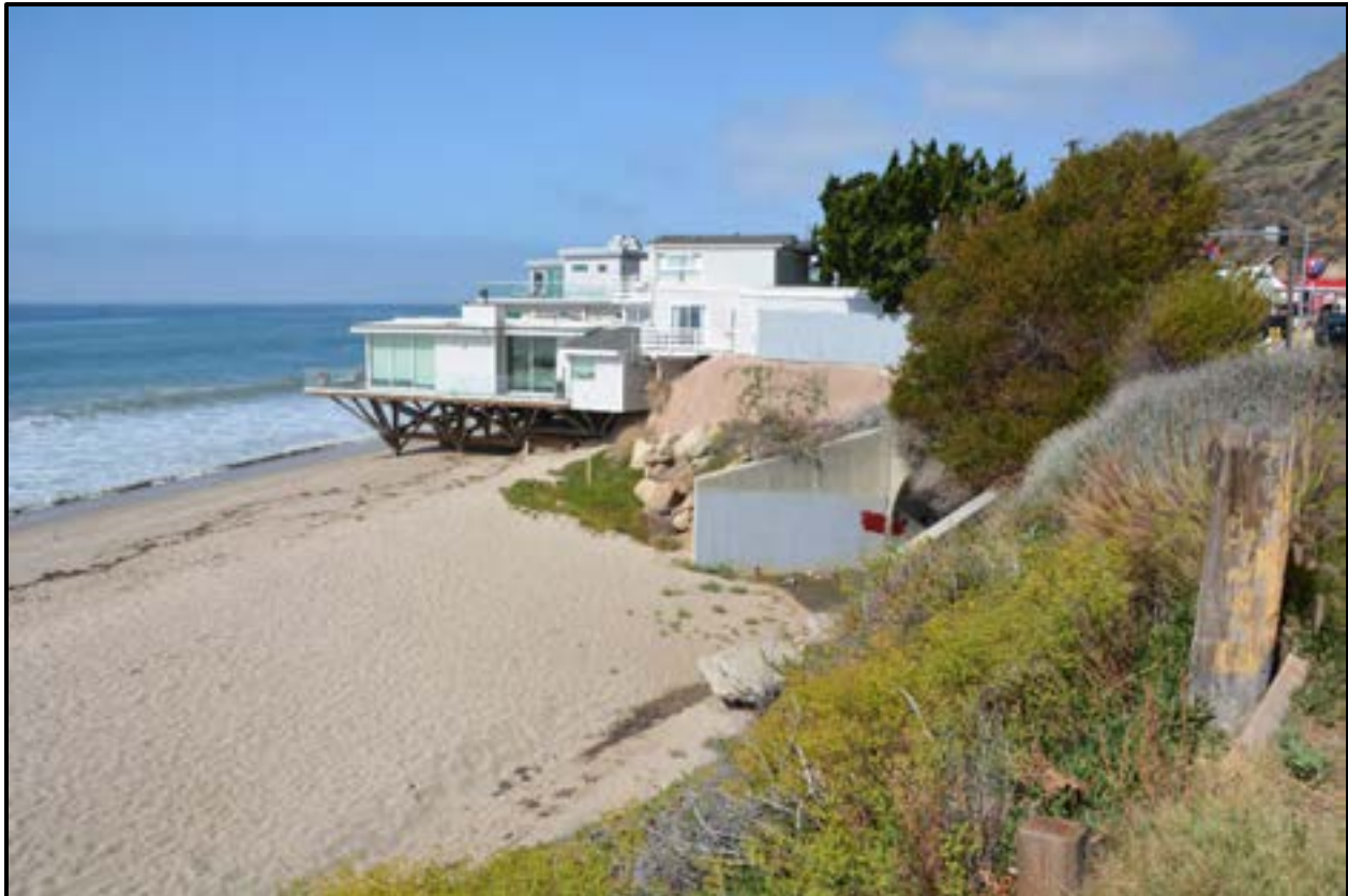
Figure 3-1. Dan Blocker State Beach downstream from Solstice Creek Culvert on May 2, 2016, following a dry period with no flow in the creek.
