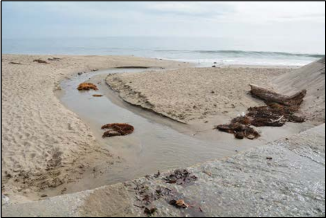
Figure 3-7. Solstice Creek, looking downstream from culvert on February 2, 2017. The creek carved out a channel with a bend.
