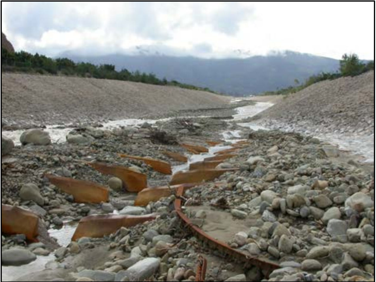
Figure 4-12. Sediment accumulation and pool damage at fish passage structure following 2004/2005 storm events in Santa Paula Creek. The creek bypassed the structure on the right bank (looking downstream).
