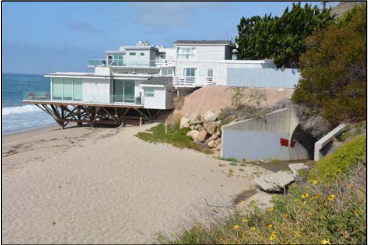
Figure 4-14. Property adjacent to culvert outlet that could be effected by increased sand buildup from any structure placed on the beach perpendicular to the ocean.
